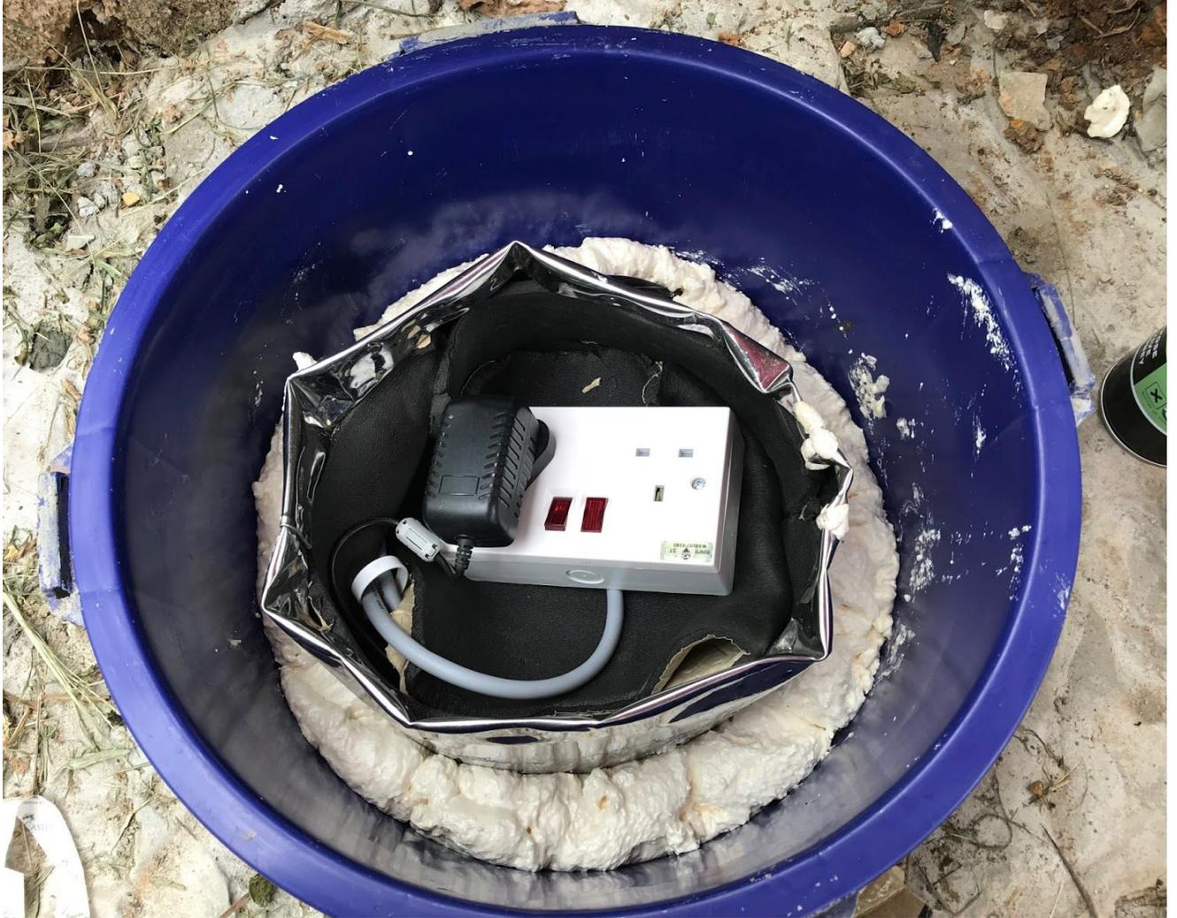
Started to place PU foam to the pail. Due to limited space, I cannot place the nozzle of the can to the base properly. Then the weather took a turn and turned bad, so I had to proceed with haste.
