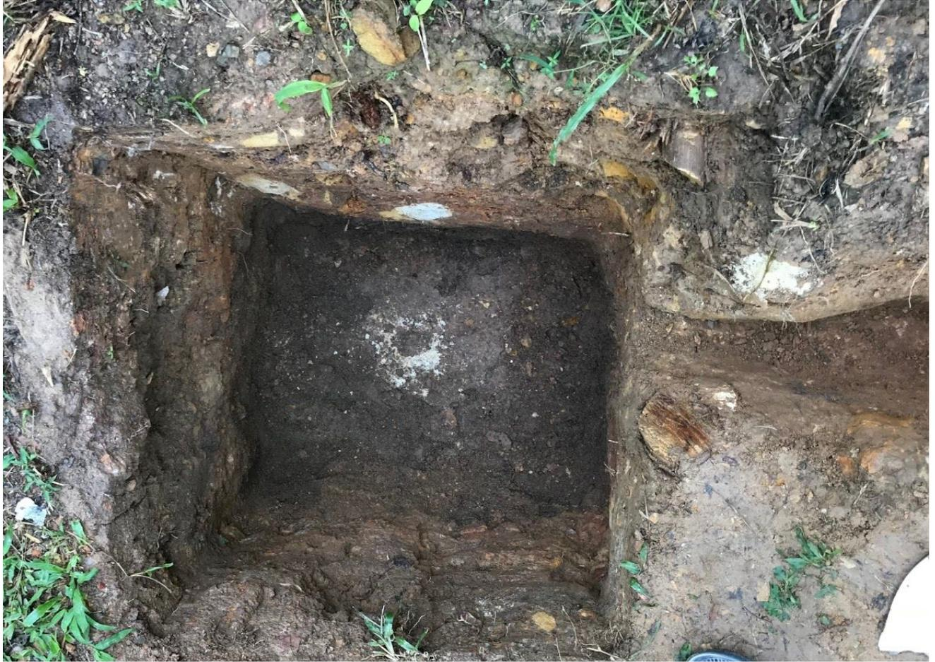
Continued work to refine the hole, remove roots and dug access for piping work for cables. Hole dimension 60cm W x 60cm L x 60cm deep (estimate). 60cm is almost 2 feet.
