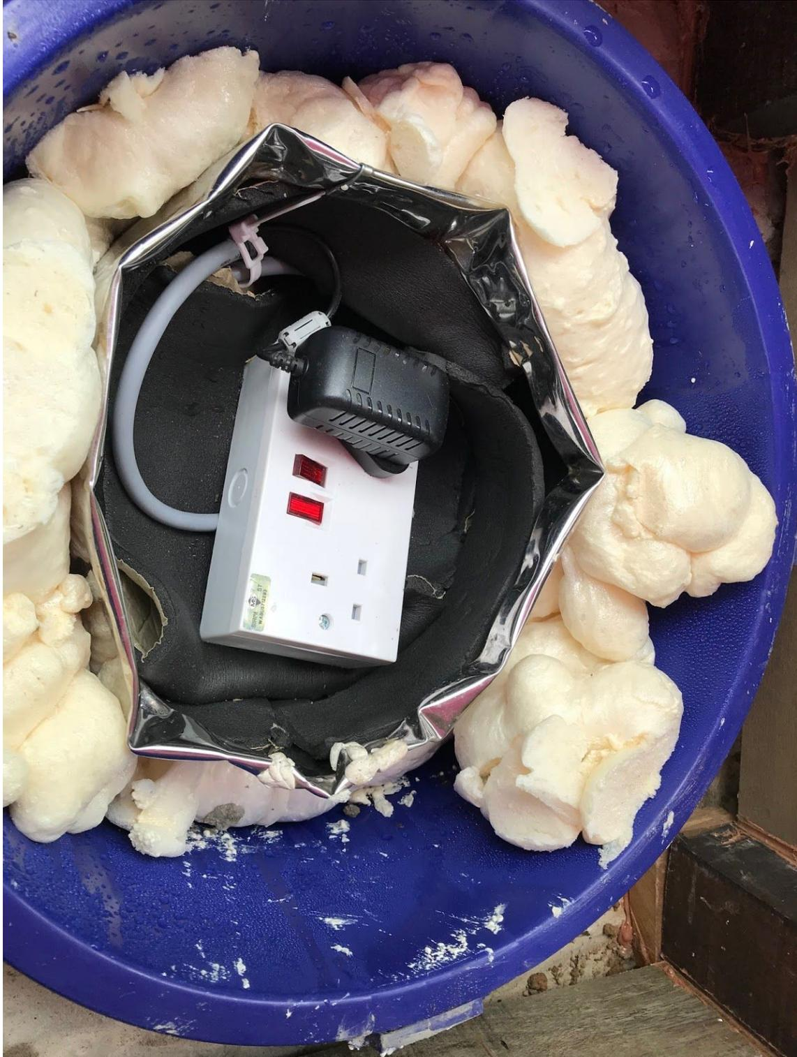
Condensation issue which is obvious - I didn't finish off the PU foam work the other day. Furthermore, the wooden enclosure wasn't airtight yet.
