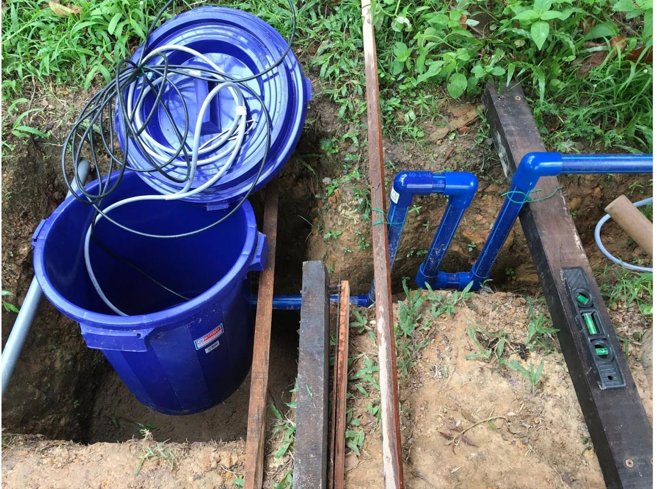
Cables pulled through and into the pail that will hold the RS4D.
