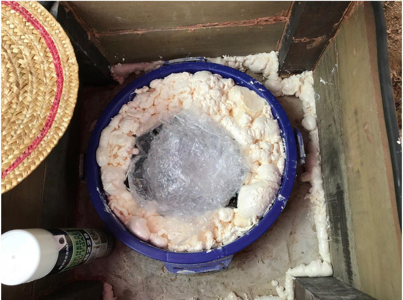
Added more PU foam and also used some bubble wrap. Wooden enclosure also ensure airtight with PU foam.
