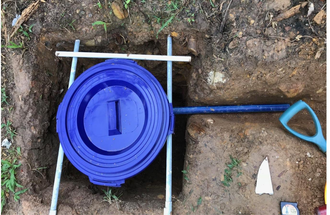
Trialing of pail positioning and also pipe for cables.
