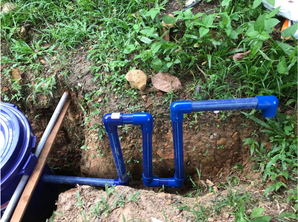
Eventual design of pipe work. I settled this to reduce any vibration from the pipe to the pail/RS4D. The bottom part will be embedded in cement. I have to say, there is no evidence to say this design is better than the simpler pipe connection. It is just something I chose in the end.
